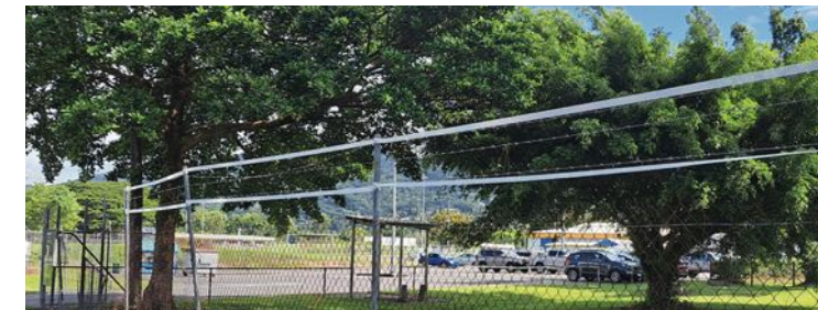
White electric fence tape and metal tags are ideal for security fences where the barbs need to remain. They move in the wind and the tags catch any light at night.
